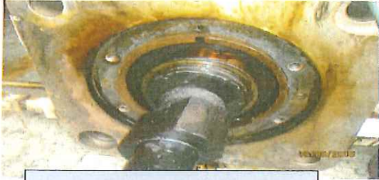
Dismantling of Fuel Pumps
